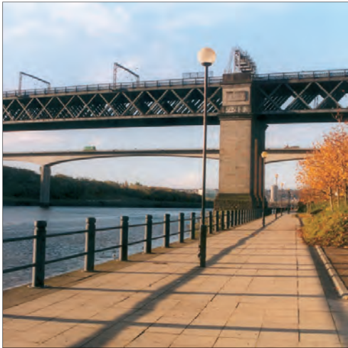
Bridges provide the main visual focus of the River Tyne
