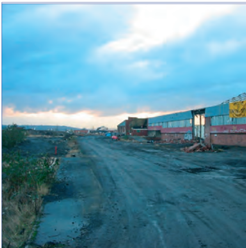
Many buildings lie derelict
