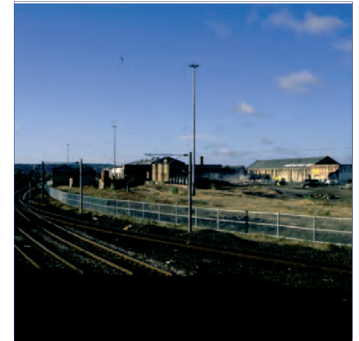
Current character is determined by the successive abandoned and derelict buildings with wide spaces between
