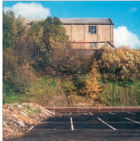
Built form is dominated by low rise industrial buildings
