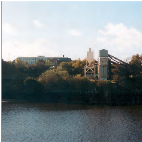
Buildings on the edge of the plateau are visible on the skyline of the Gorge
