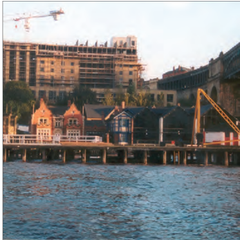
Remnant buildings at the southern bridgehead of the Swing Bridge present a colourful facade
