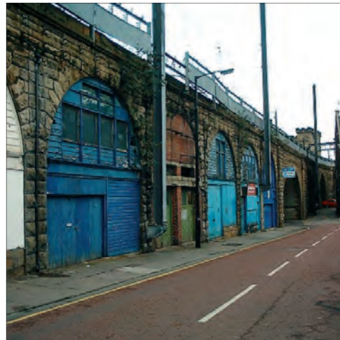
Railway arches are used as workshops
