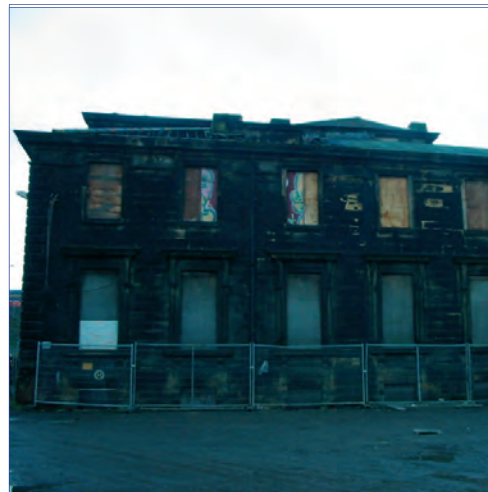
Historic stone buildings are worthy of conservation
