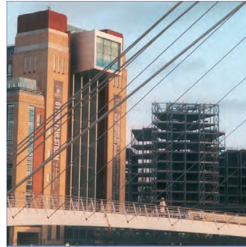
The Baltic flats (currently under construction) do not detract from the landmark Baltic Mill
