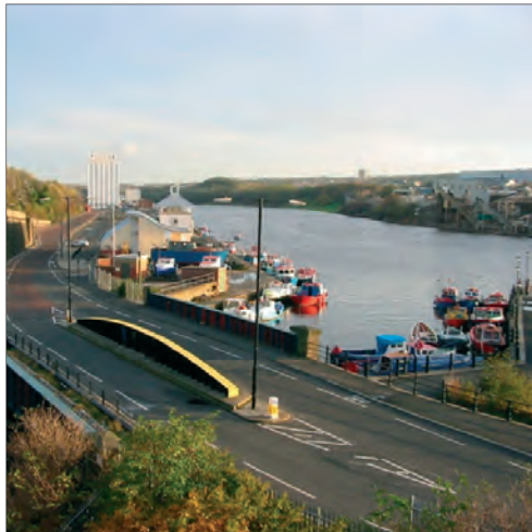
View along St Lawrence's Quayside from the mouth of the Ouseburn. Showing the Ouseburn Watersport Centre with Spiller's Mill beyond
