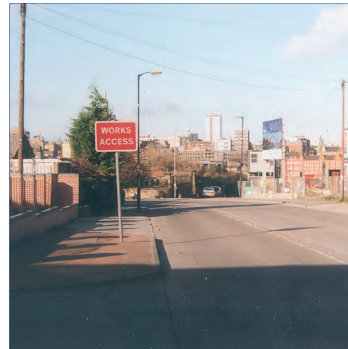
Demolition of historic buildings has resulted in loss of enclosure and sense of place
