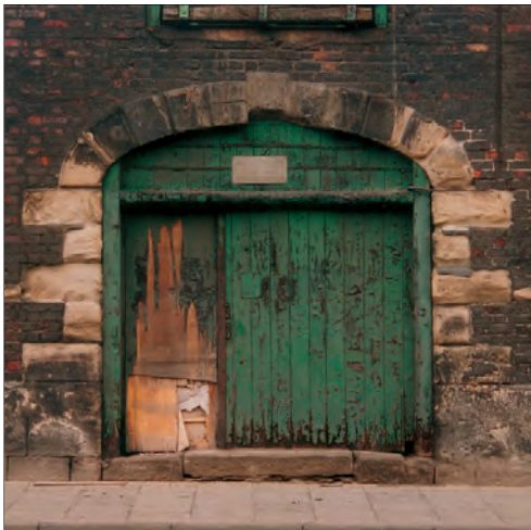
Sandstone detailing on brick warehouses
