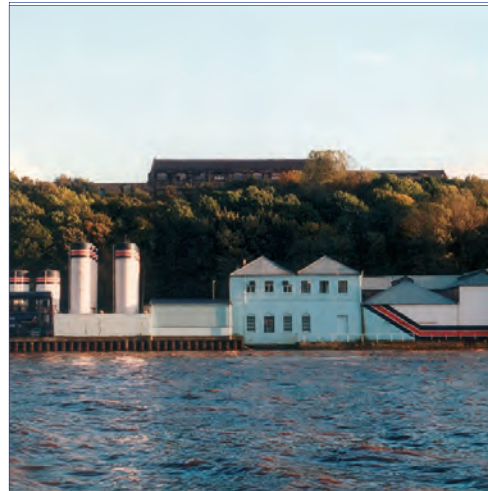
Railway works buildings are visible on the lip of the Gorge
