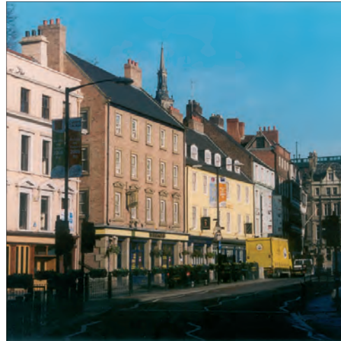
Coloured render on buildings along Sandhill enlivens the street scene
