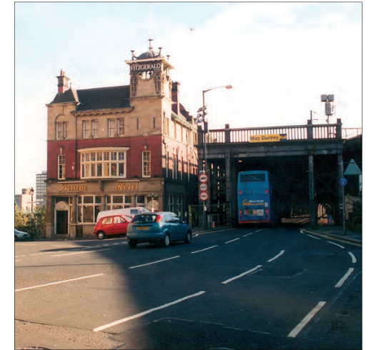
The High Level Bridge extends across the Gorge from this area
