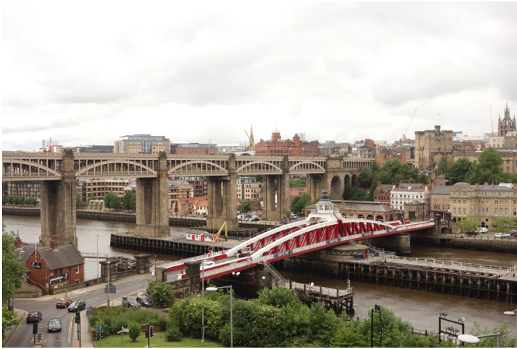
High Level and Swing Bridge
