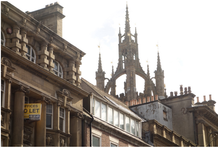
Chimney pots and Crown Steeple off Mosley Street
