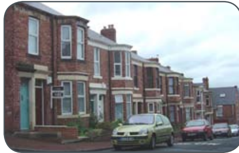
Double-height bay windows distinguish these later examples of the Tyneside Flat
