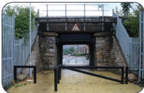
Armstrong Street underpass
