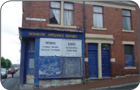
Corner shop unit, Balfour Street
