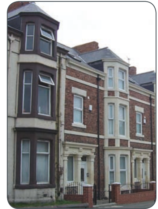
Whitehall Road before and after refurbishment and conversion
