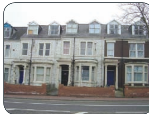
The high profile of the old Great North Road meant the buildings on the Durham Road corridor were built on a grander civic scale - they are now enjoying refurbishment after a long period of decline and blight by traffic. This will improve perceptions of the neighbourhood.
