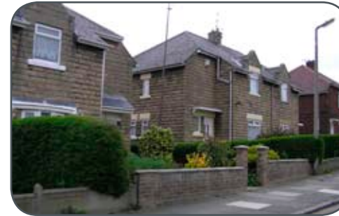
Inter war garden suburb style council housing on the Field House estate
