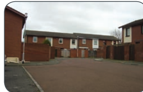
Poorly integrated public environment in Radburn layout estates to the north of the area
