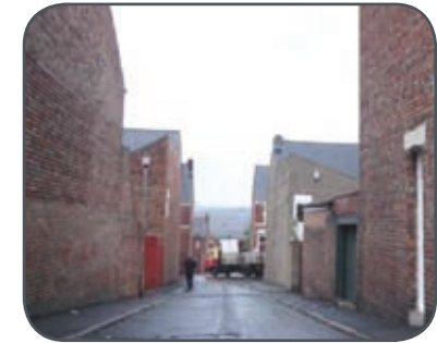
Blank gable ends on east-west routes
